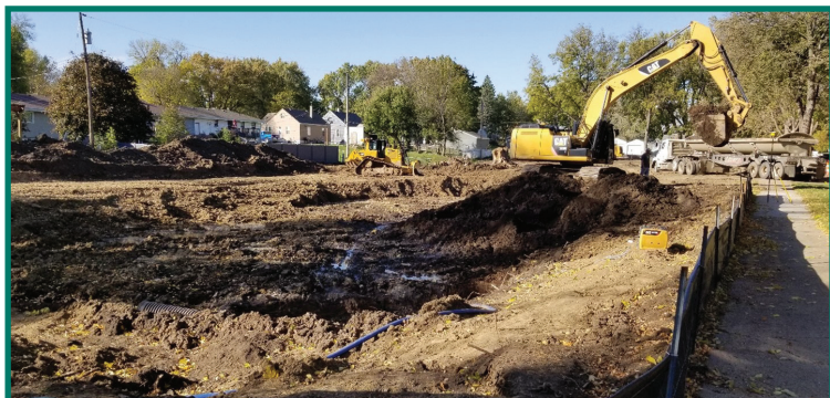
Initial grading and excavation of the bioretention cell began in October 2021.
