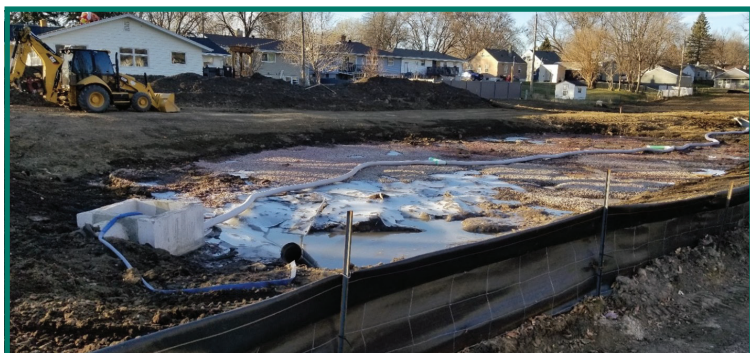
Underdrain and stormwater infrastructure install in November 2021.
