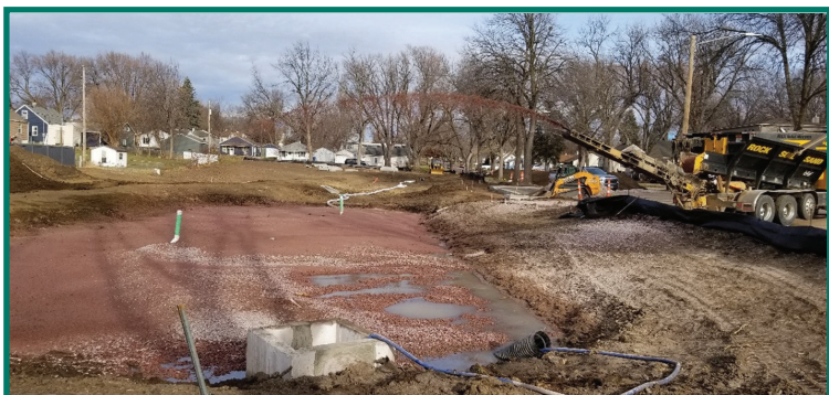
Bioretention cell media installed during December 2021. Note the installation technique. Care was taken to avoid heavy equipment compacting media within cell.
