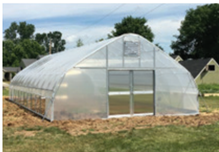
Figure 1. A traditional gothic style high tunnel.
